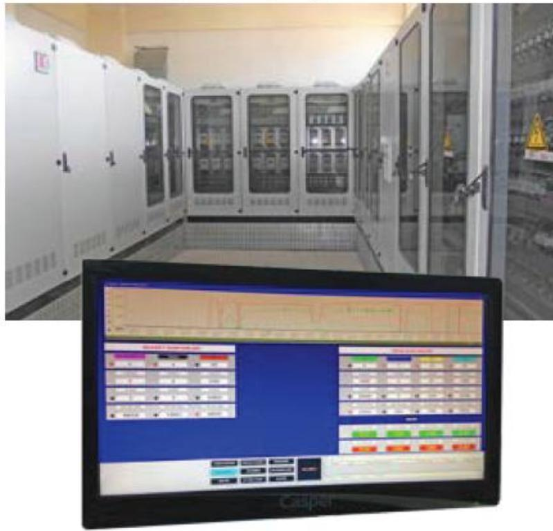
Electrical and automation works for wheat flour and semolina mills and feed mills, design and manufacturing of MCC panels; design and manufacturing of compensation panels; PCL programming & SCADA software; erection of field cable trays. Yield, humidity and flow control systems.
