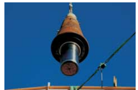
Main Shaft being installed
