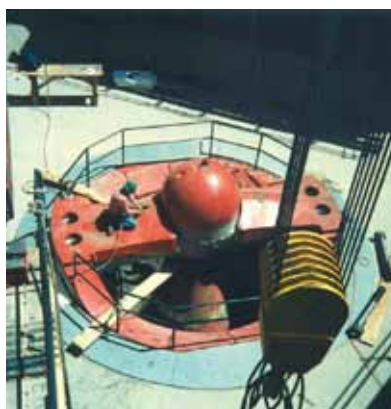
Installation of Primary Gyrator
